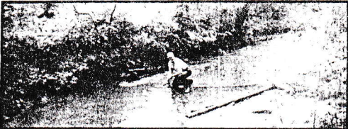
Bill Kelly is kneeling on a deflector he helped build. It runs from the near bank out to Bill and shoots water against a cover log on the far bank. Last year this was just a flat, sandy pool devoid of cover or food. Now it has a gravel bottom and fat, native trout.
