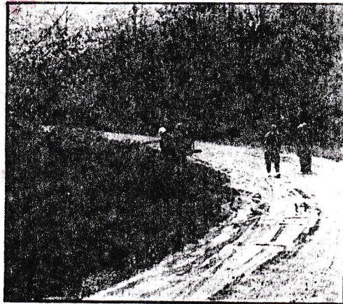
Most of us would consider this a good mountain road. But this road has destroyed 4 1/2 miles of a native trout stream.
