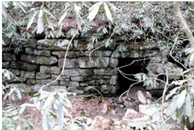
Stone Culvert for Dick's Creek beside the Sandy Ford Road
