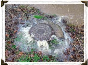
March 4, 2008: This picture shows raw sewage flowing directly into Scott Creek (the west prong of Stekoa Creek) from an overflowing City of Clayton sewage collection system manhole. Yes, a little bit of rain does make a big difference. But why? Does the rain saturate the soil and infiltrate failing pipes and joints, causing the sewage collection system to overflow?
